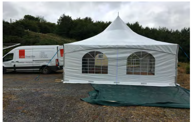
Our 6m x 6m under construction in Innishannon for a home wedding. 40 guests attended. Side-view. Flooring installed. July 2021.
